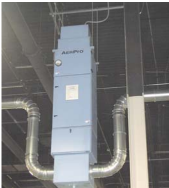
VOMC 3000 with HEPA on automotive oil mist stands
